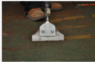
Ship Deck Rust Removal
