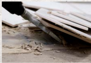
Ceramic Tile Removal
