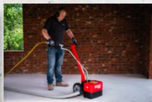
Fast Removal of Concrete
