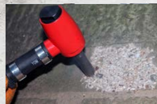
Reducing Levels on Concrete
