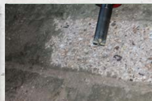
Roughening Concrete
