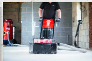
Removing High Spots
