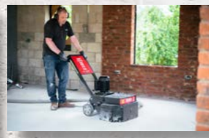
Grinding Concrete
