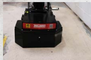
Polishing Concrete Floors
