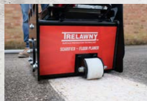
Reducing Levels on Concrete
