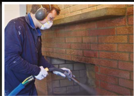
Wood and Brick Cleaning
