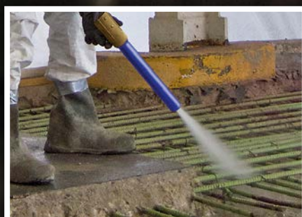
Concrete Repair and Restoration
