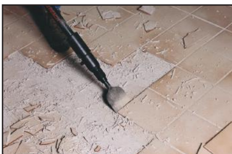
CERAMIC TILE REMOVAL
