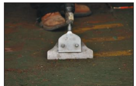
SHIP DECK RUST REMOVAL
